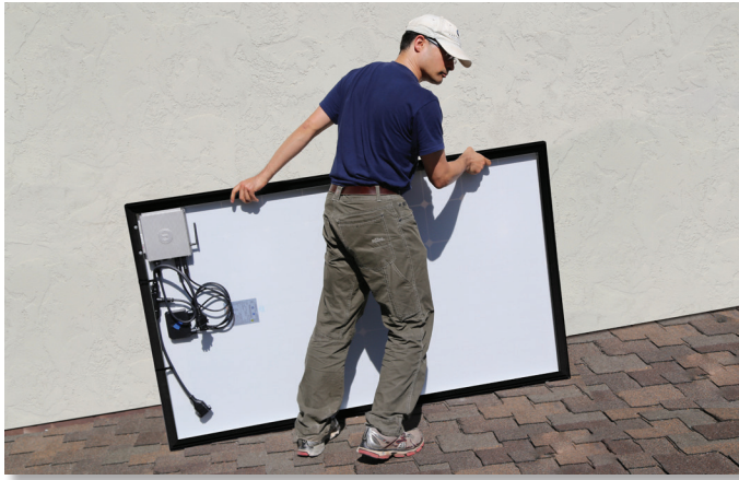
Bottom View of Panel Assembled with Microinverter
